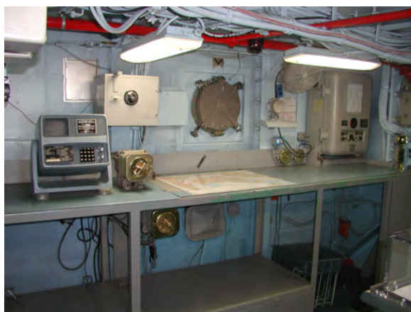
Port Bulkhead with Chart Storage Below
