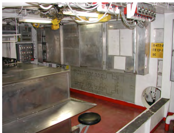
Telephone Talker Station (Foreground)
