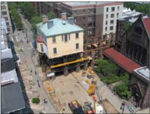
Photo courtesy of www.wolfhousebuildingmovers.com Alexander Hamilton's "Country House," built 1802, is lifted to be moved around a church in New York City (2008).
