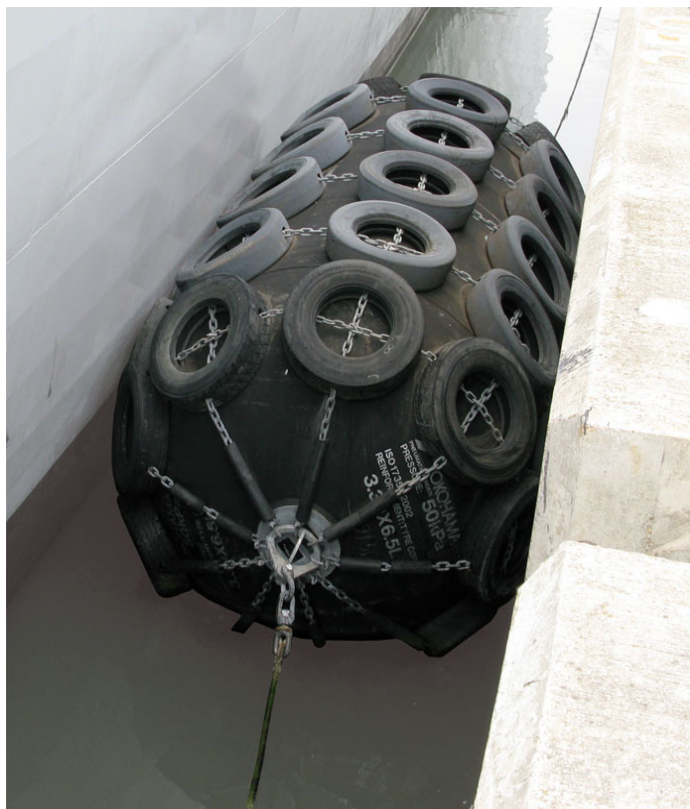
Fig 3-219. Port Fendering – Large Pneumatic Fender
