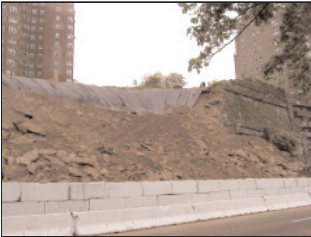
Safety blocks installed to protect roadway.
