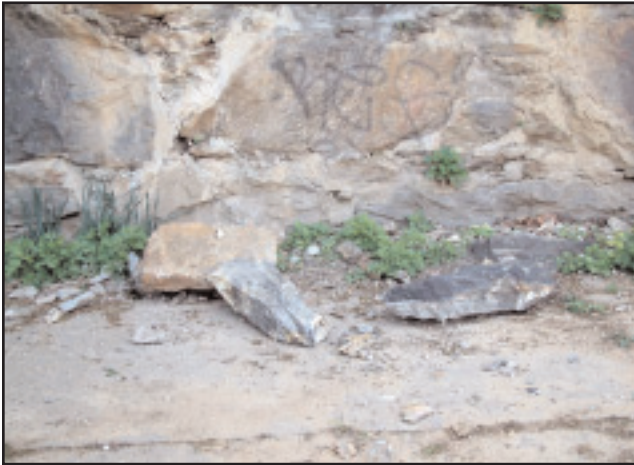
View of fallen rocks on May 9, 2005.
