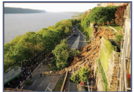
Castle Village Retaining Wall Collapse April 2007
