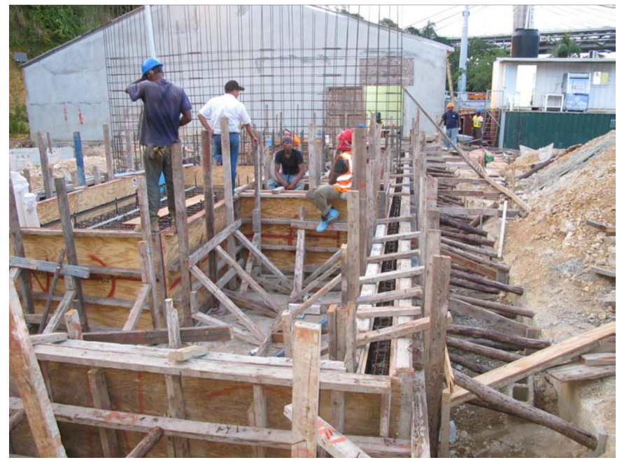
Foundations for Towers & Transformers
