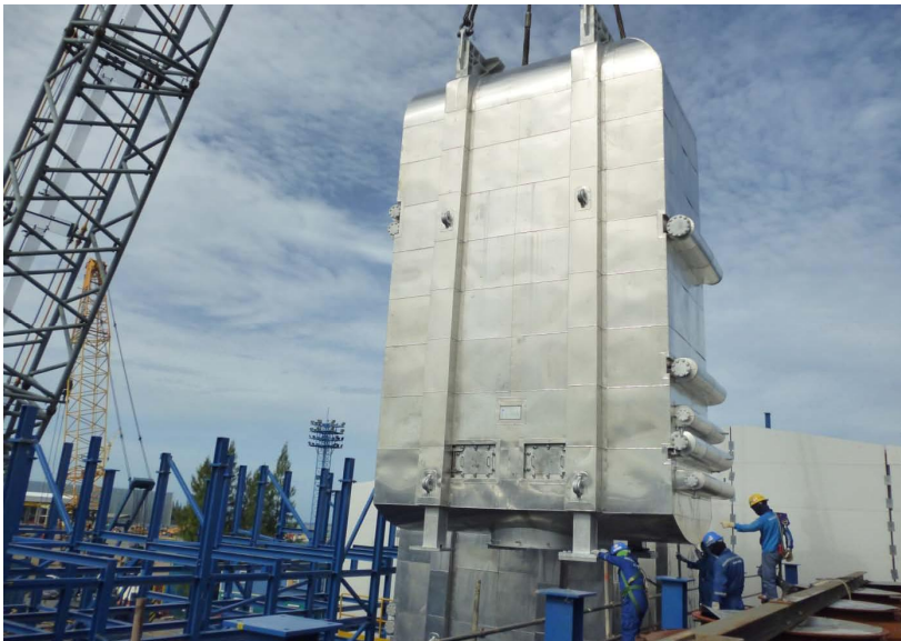
Exhaust gas boiler installation (1 of 6) 7/16/2011
