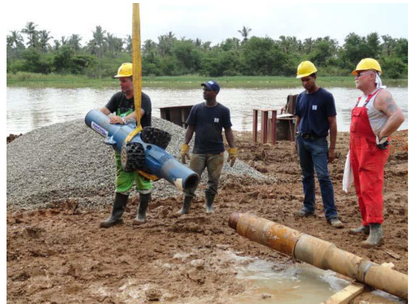
Reamer to increase from 8" to 20" diameter
