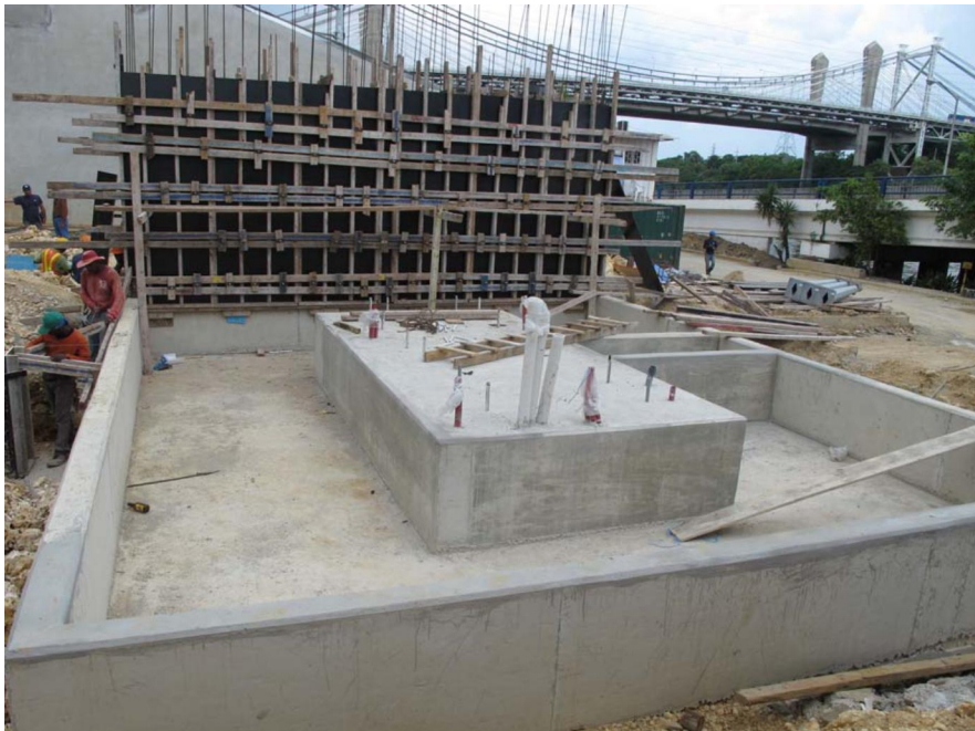
Step-up transformer base and oil collecting pit
