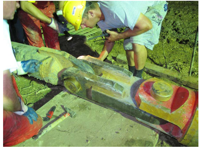
Swivel connected to gas pipe
