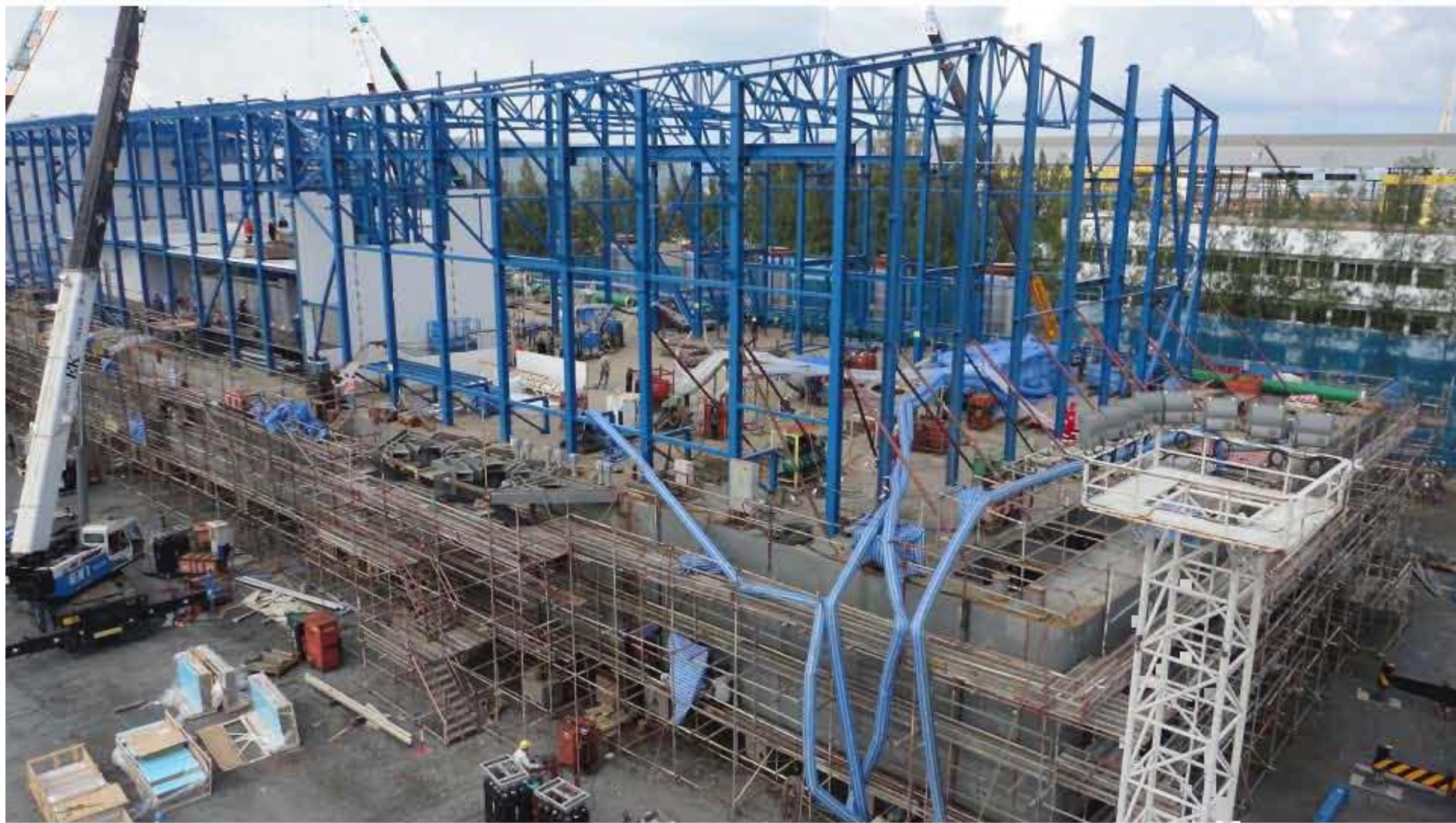
Construction of Power Plant Housing Structure - May 27, 2011 The structure can withstand wind speeds of up to 120 mph for one minute
