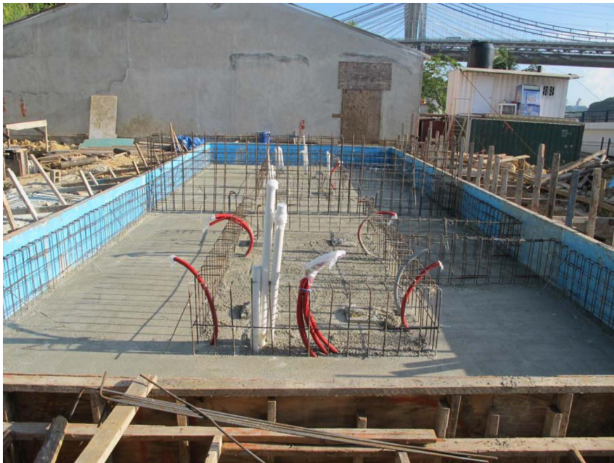
Foundations for Towers & Transformers
