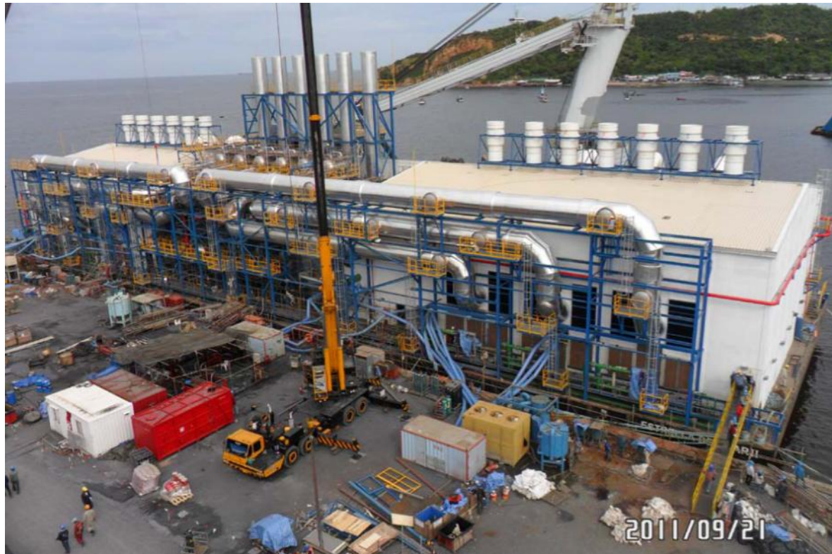
View Starboard Side (Without scaffoldings) - Note finished exhaust ducts & HR system.
