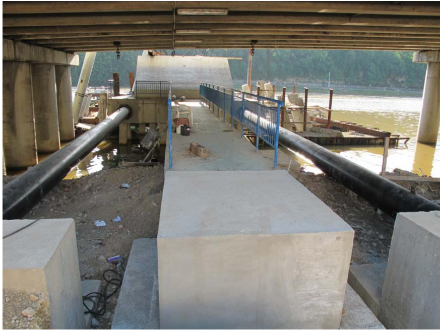
Connecting piles with steel beams and casted concrete (yellow gas pipeline)
