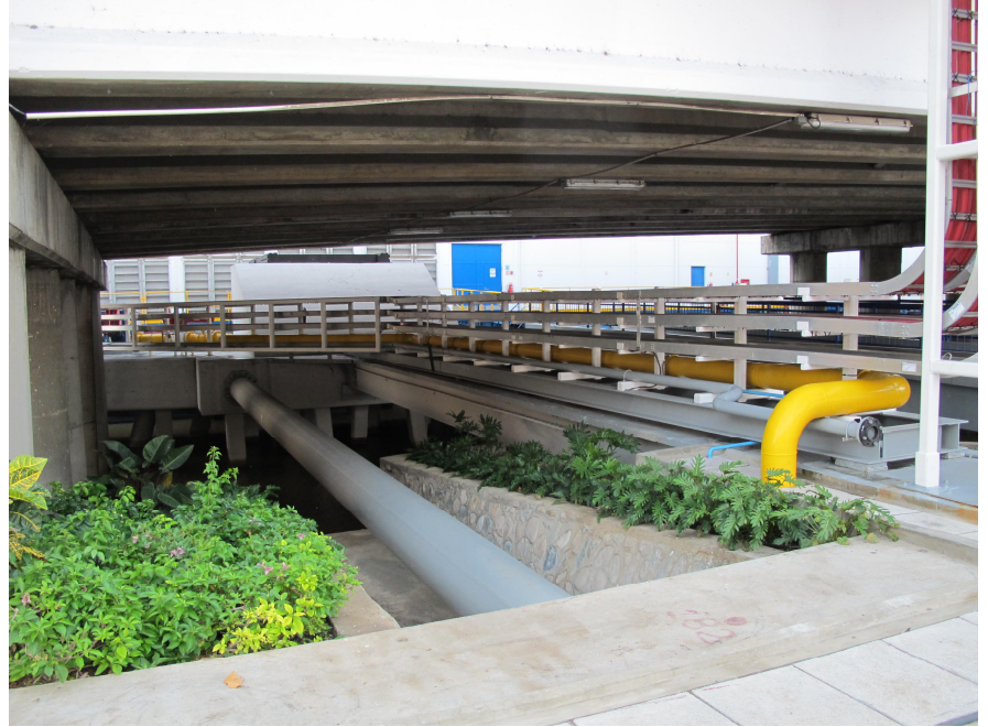
Connecting piles with steel beams and casted concrete (yellow gas pipeline)
