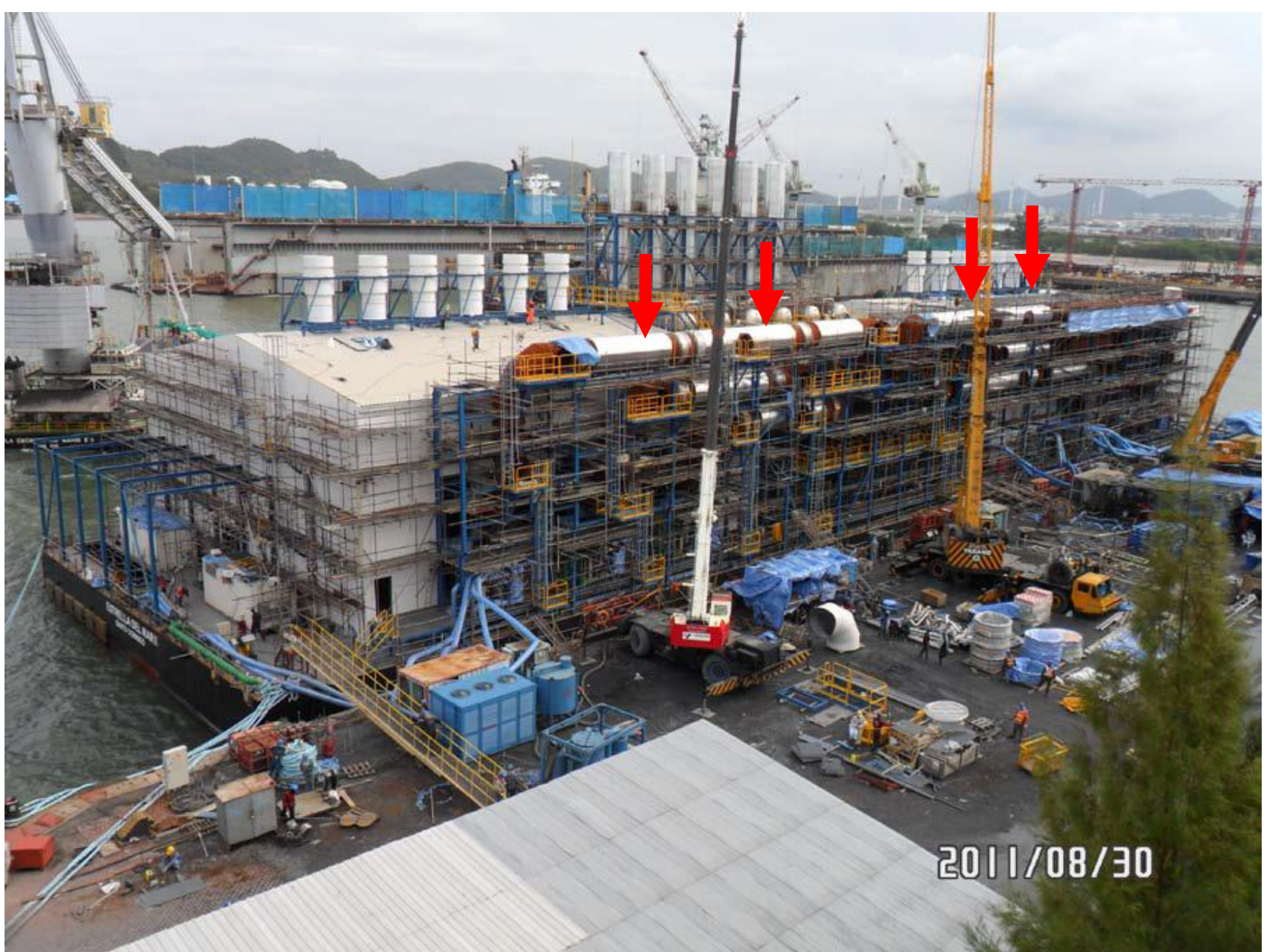
View Starboard Side – Initial work on exhaust ducts from each engine for heat recovery system, which cannot be directed out as usual, but have to be turned inward, with the boiler and the stack area located in the center.
