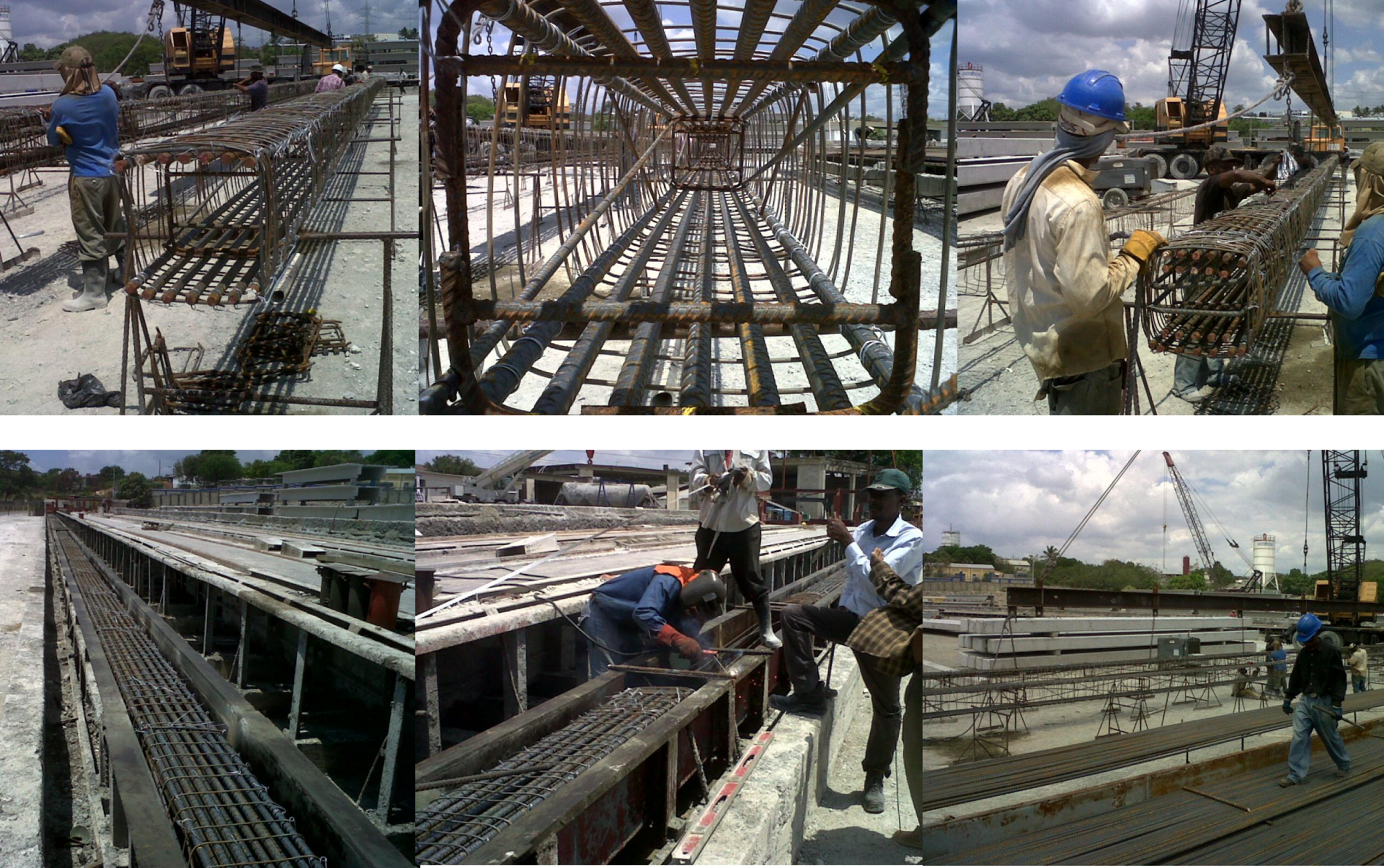
80' long piles were used to reinforce the existing moorings
