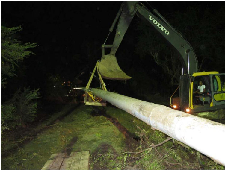
Pipe lifted (to provide angle) and on rollers
