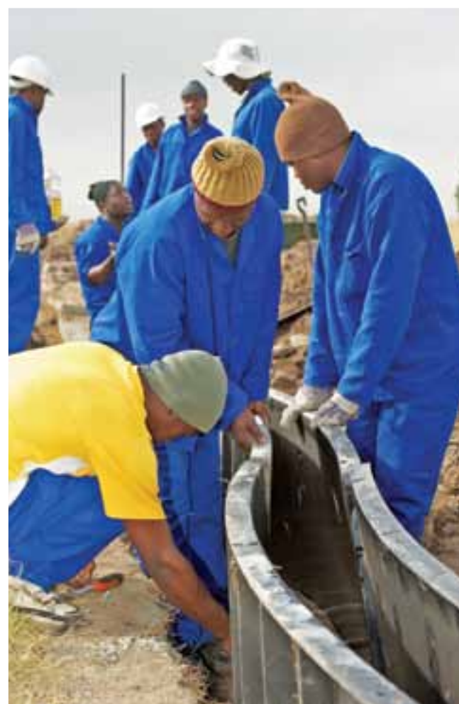
The first section of the framework being laid on top of the foundations.
