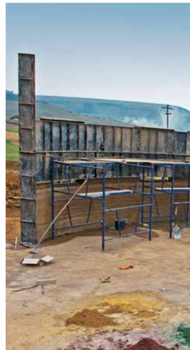
Construction of the first wall section under way at Mampunga Primary School.
