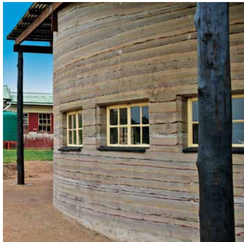
The new rammed earth classroom block at Buhlebamangwe with the old building it is replacing in the background
