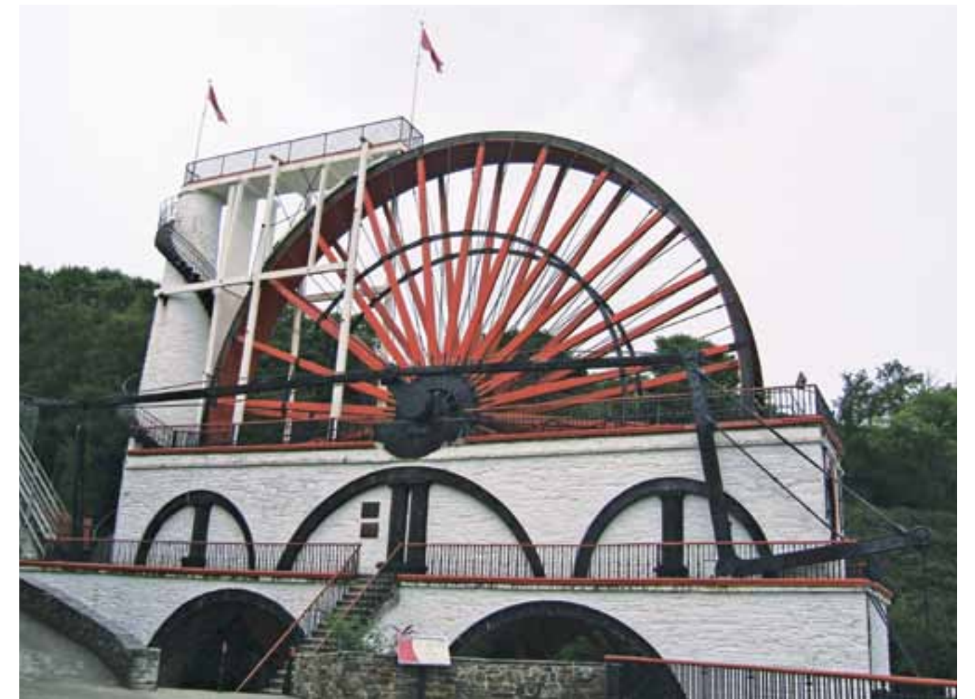
Laxey Wheel, the biggest mine pump waterwheel in the world.
