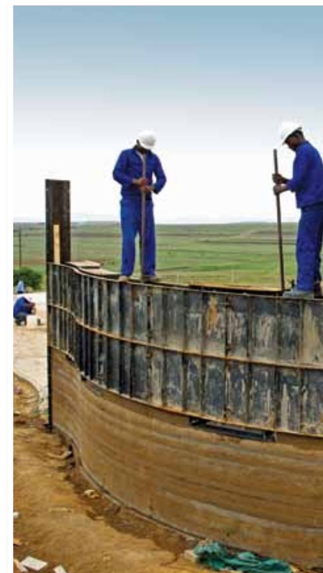
The labour intensive 'ramming' produces a permanent and low-cost structure. The lines of ochre add some colour to the otherwise grey walls
