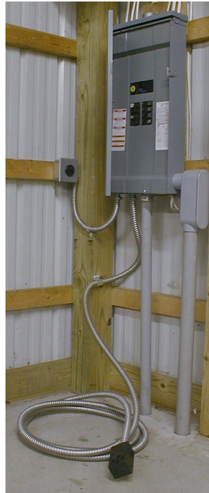
Figure 70: I have my panel wired with a wall mounted 240v receptacle, and this "drop lead" receptacle that allows me to move the welder about the shop.
