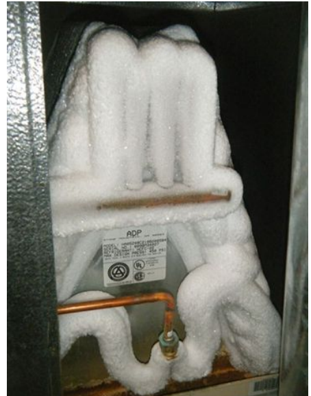
Figure 2 Frozen Coils
