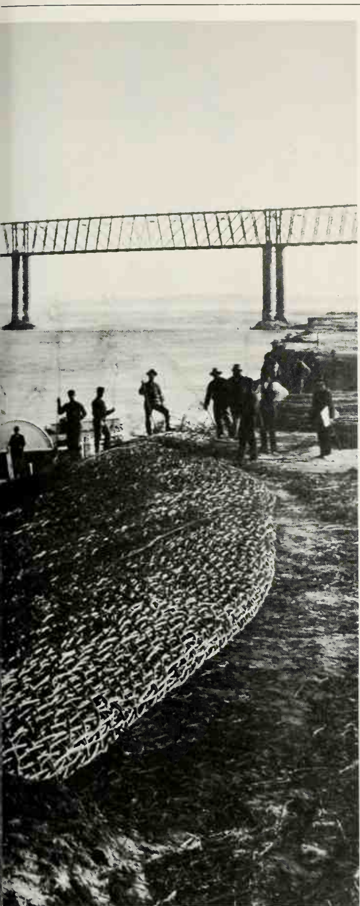
designed to arrest cave-ins along the bank. Boulders anchored it in place.
