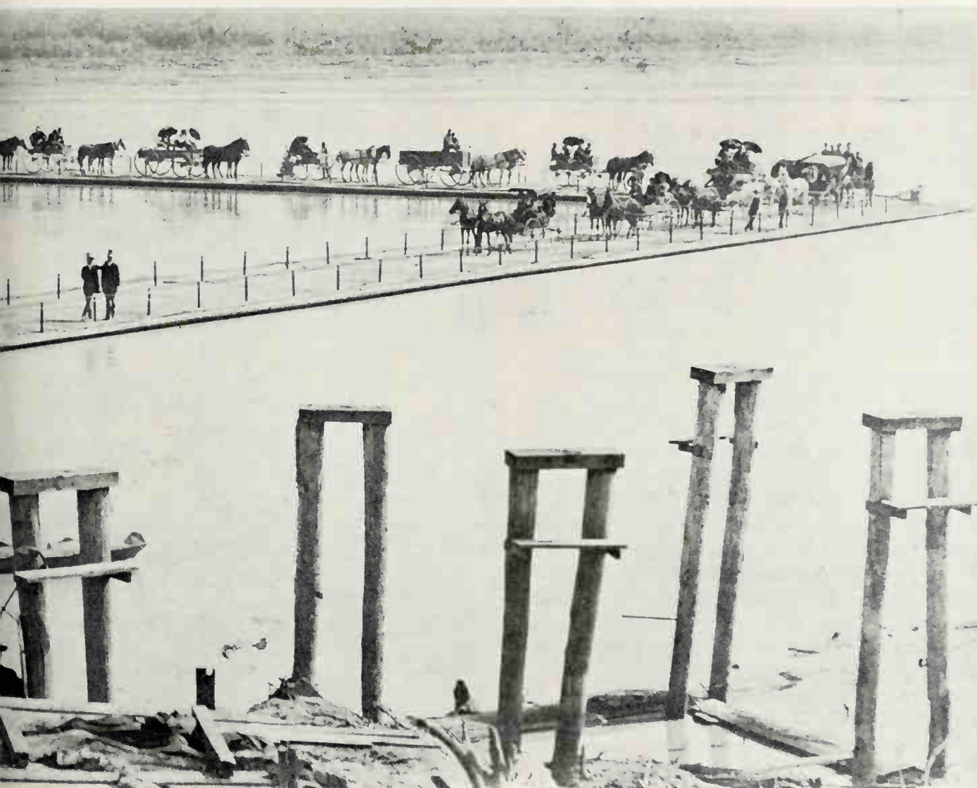
structure was designed to part at the point of the V to permit the passage of steamers. A flood wrecked it after only four months of service.
