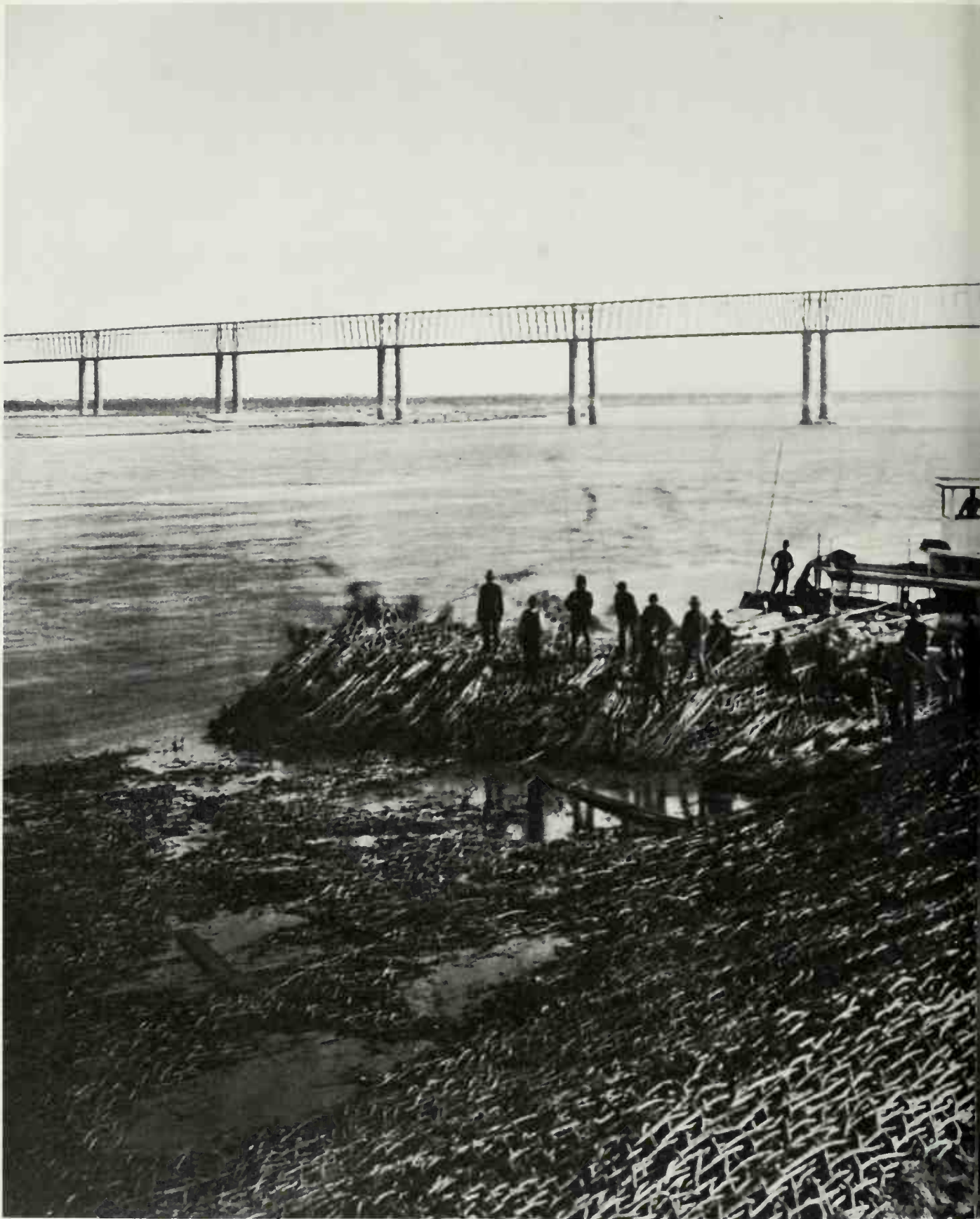
Near a railroad bridge at Omaha in 1880, U.S. Engineers, supplied by steamboat, supervise the weaving of a huge retainer made of saplings and
