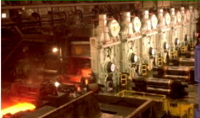
Finishing mill Fire brigade Fire detection
