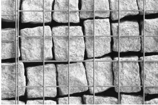
FIGURE 12.31 Gabion basket wall.
