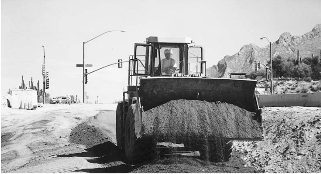
FIGURE 3.1 A highway under construction.
