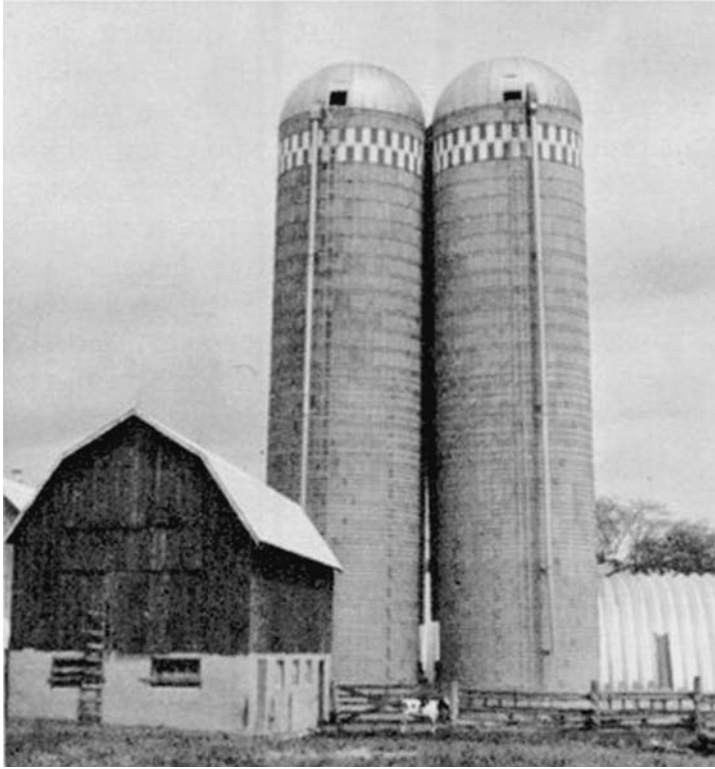
FIGURE 5.1 The “kissing” silos (Bozozuk, 1976, permission from National Research Council of Canada).
