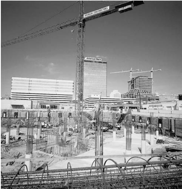
FIGURE 10.1 Concrete piles used for the foundation of a skyscraper. (© Fritz Henle/Photo Researchers.)
