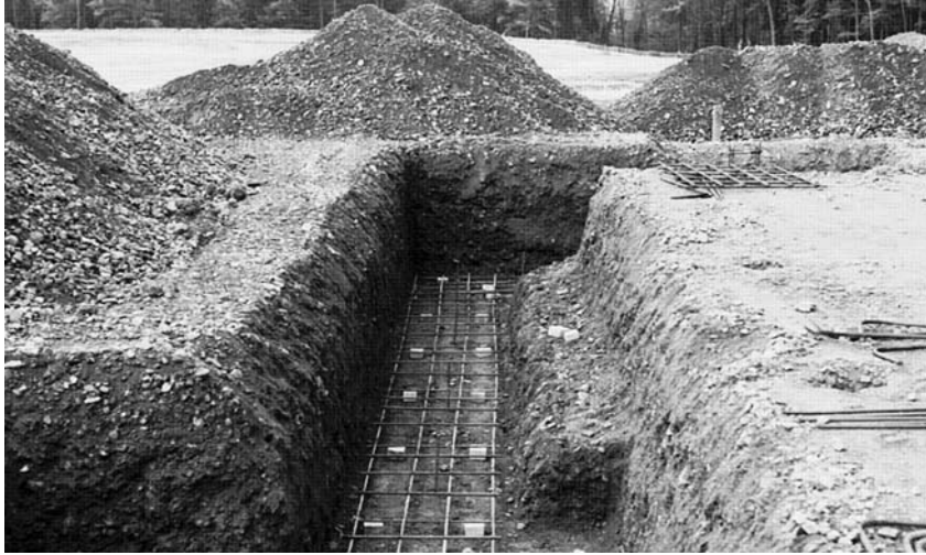
FIGURE 9.1 Construction of a shallow foundation.
