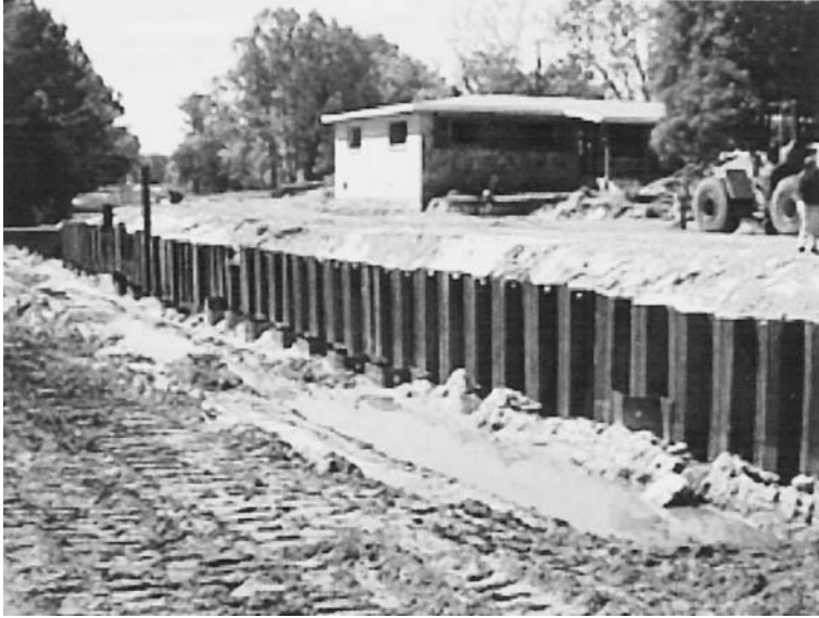
FIGURE 12.1 A flexible retaining wall under construction.
