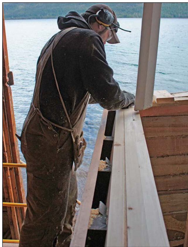
With DeSMET’s boathouse doors open to the lake, one of Burch’s staff sands the new railcaps.
