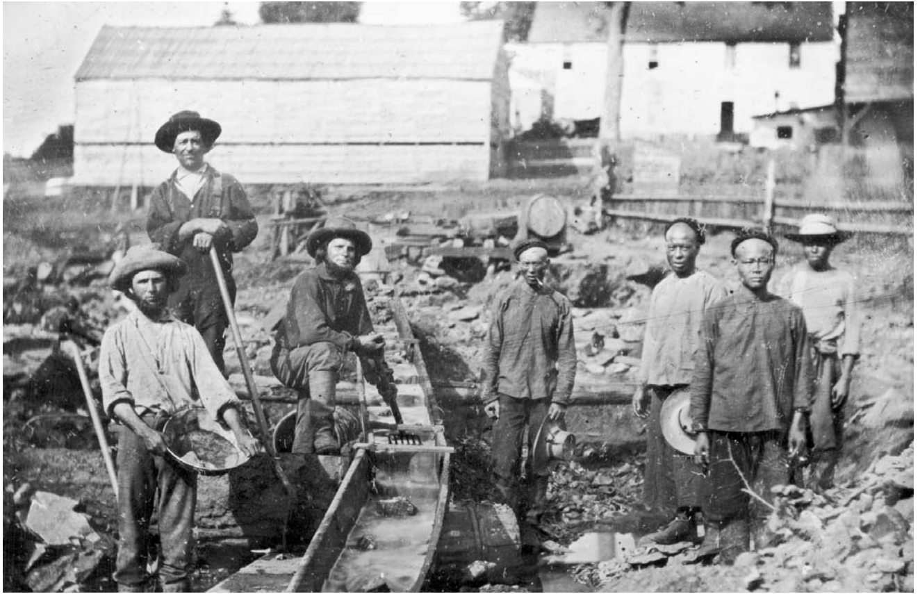
Chinese miners stand next to a sluice box, Aubine Ravine, California, ca. 1852. (Fotosearch/Getty Images)
