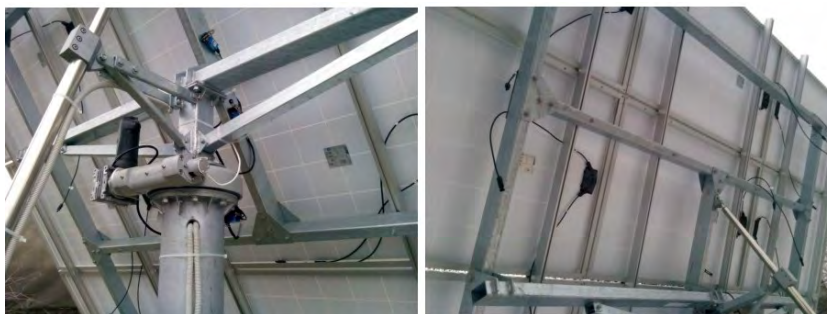
Figure 21.10 Combined linear drive and rotation drive pan-and-tilt sun tracking system to change the angle of a solar panel array (SolarTech, 2014).
