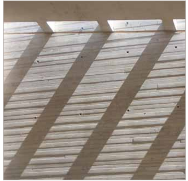
Board-marked in-situ concrete at The Collection, Lincoln.
