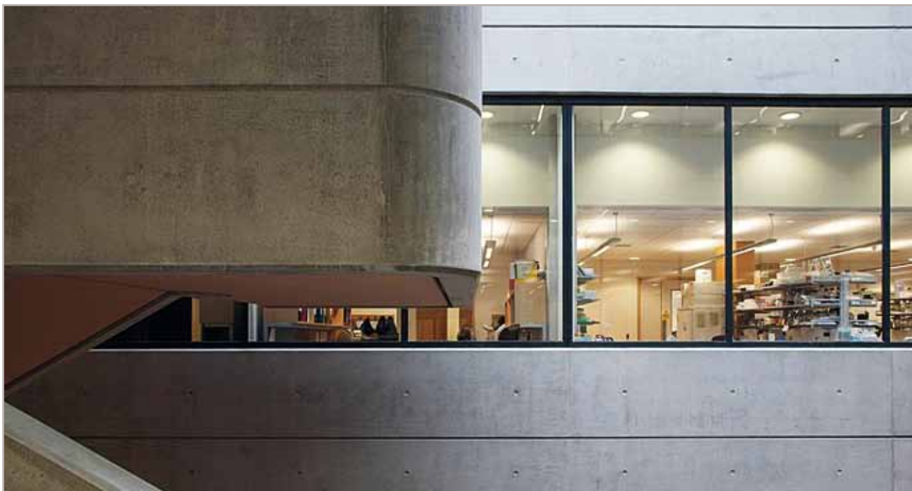
Recess detail at construction joint between wall and floor at Old Road Campus Research Building, Oxford.
