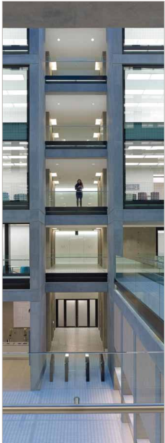
Visual in-situ concrete, incorporating cementitious binder with 34% fly ash, at the Angel Building in London.
