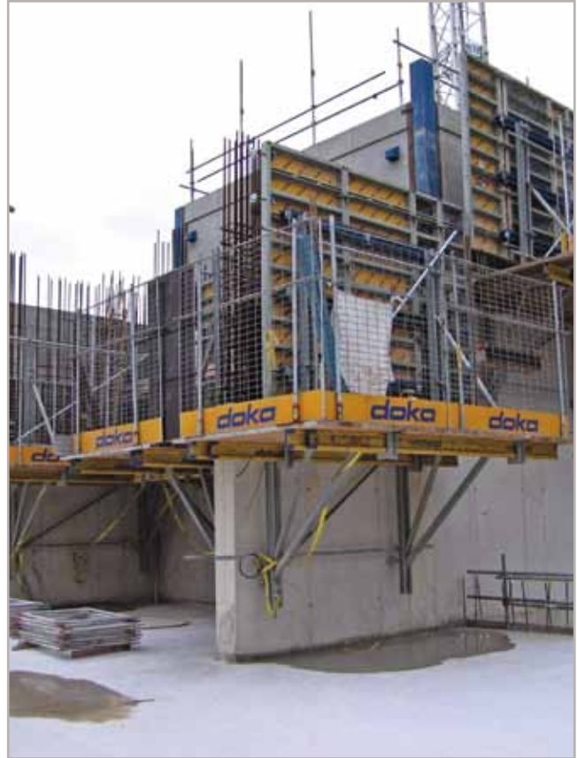
Formwork panels at One Paradise Street, Liverpool. Courtesy of DOKA.
