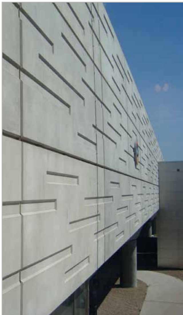
Precast concrete cladding used at Shoreditch Station, London.
