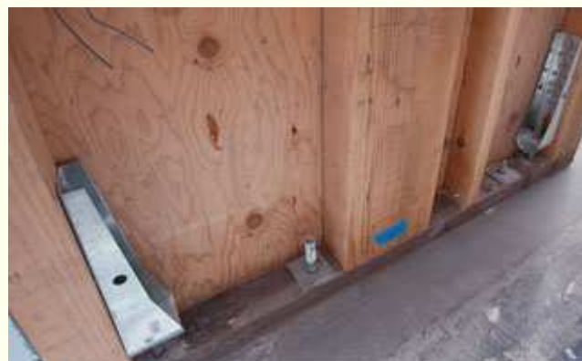
Anchoring to the foundation.
