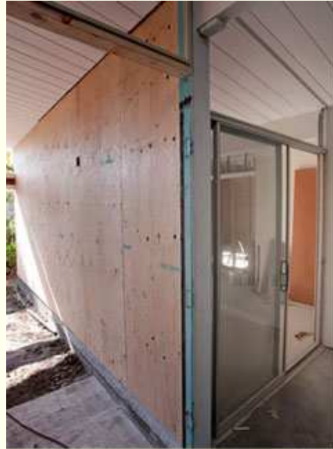
Shear wall bracing.
