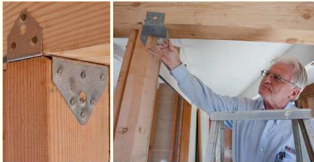
Ron Key of Keycon, Inc. demonstrates a metal post-and-beam bracing connection, one of the earthquake retrofitting reinforcements he recently installed in a peninsula Eichler.
