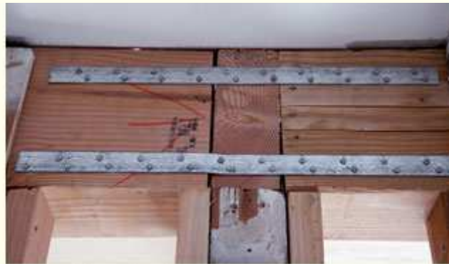
Post-and-beam bracing.
