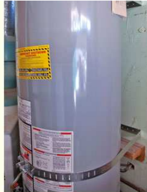
Water heater strapping.
