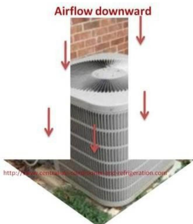
Airflow upward is efficient and logical to me. Here is my reason for that. Over the year, leaves, debris and dirty tend to be inside the condenser units. If the air conditioner fan were to force air downward, it would force the foreign material into the aluminum coil and trap it there.
