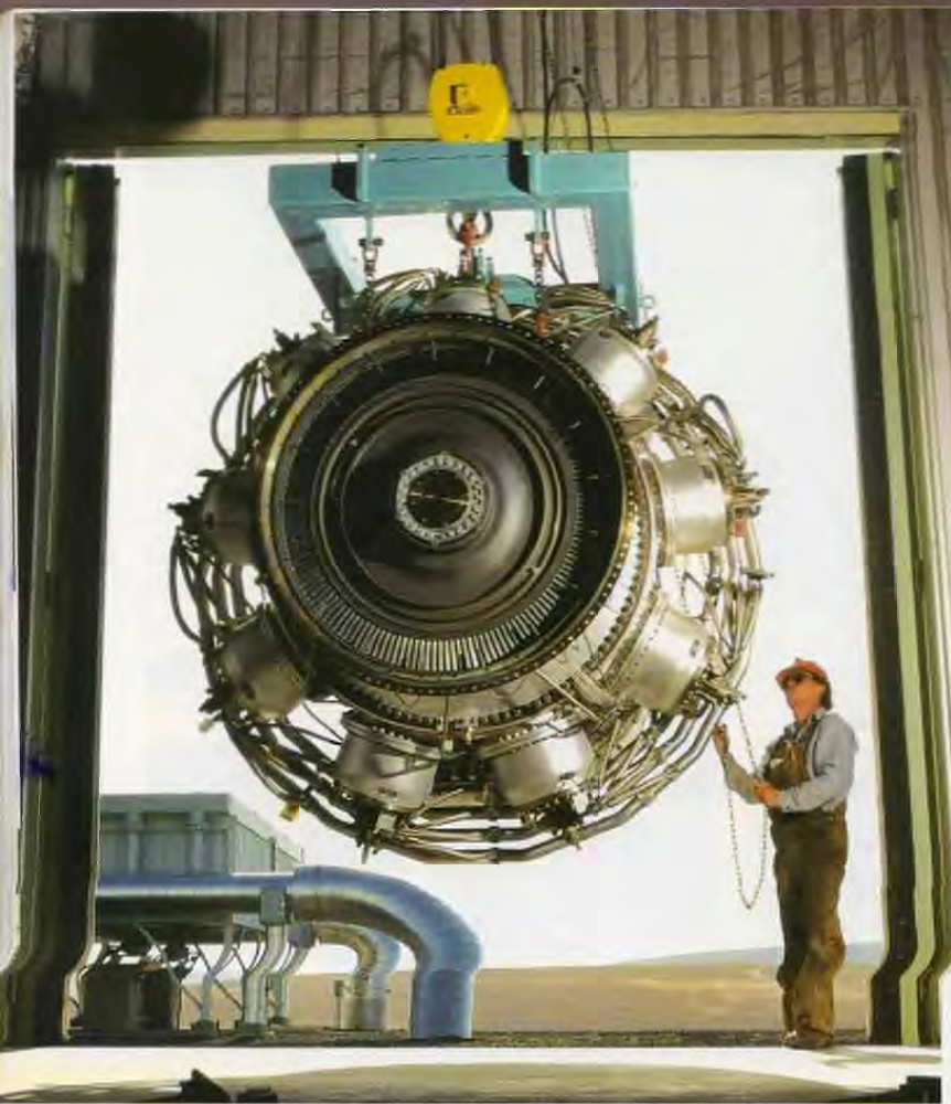
Industrial RB211 being installed
