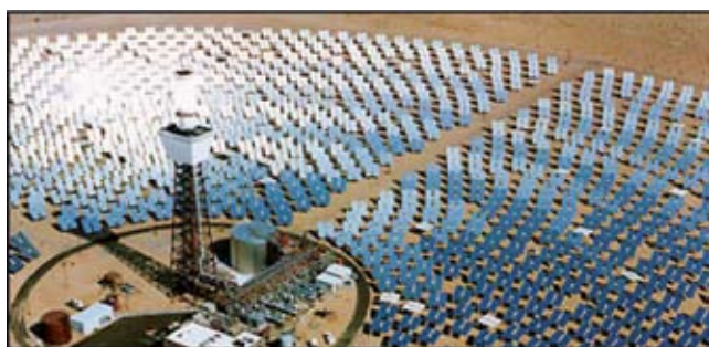
Figure 10. Solar 2 power tower in Barstow, California. The plant uses a combination of 60% sodium nitrate and 40% potassium nitrate as a working fluid and heat storage medium.
