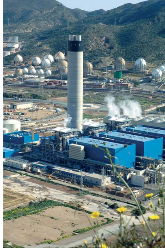
The completed 1200 MW Cartagena plant
