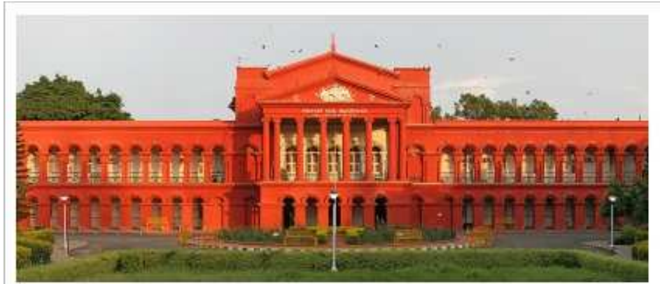
Originally Attarakacheri now the High Court of Karnataka in Bangalore at the entrance to Cubbon Park
