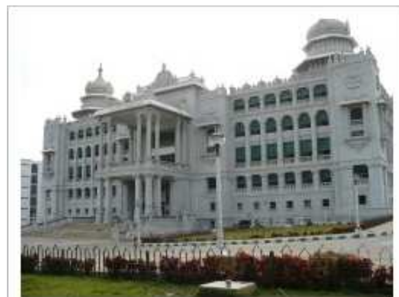
The Vikasa Soudha, situated adjacent to the Vidhana Soudha, houses many state ministries.
